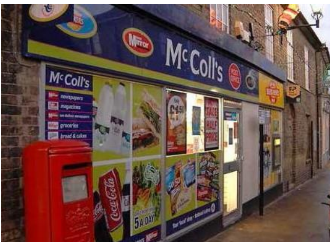
Window stickers can dominate and deaden a shop frontage
