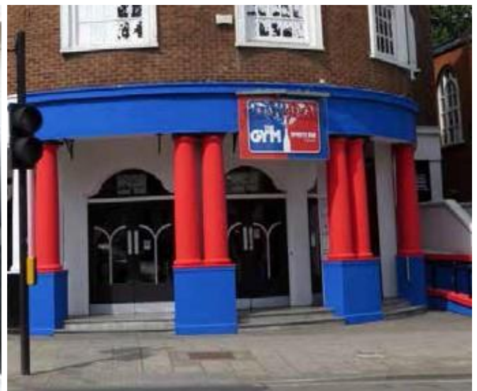
Inappropriate use of visually dominant colours
